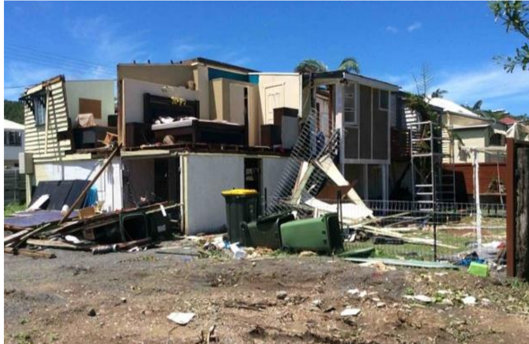
Wind, flood damage in Yeppoon, QLD
